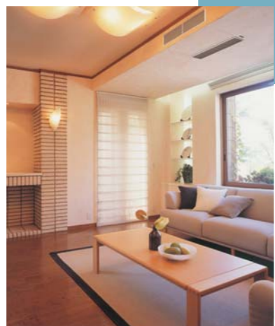
Only 240 mm is required above the ceiling for installation.
